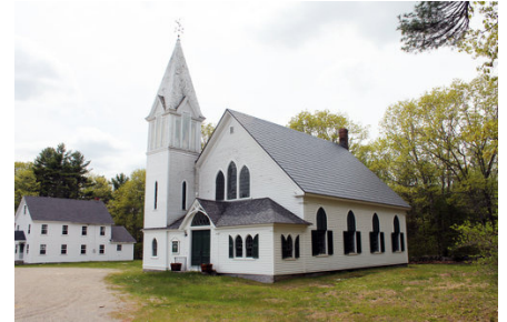
Bunker Hill Baptist Church 1185 Bunker Hill Road Jefferson, Maine
